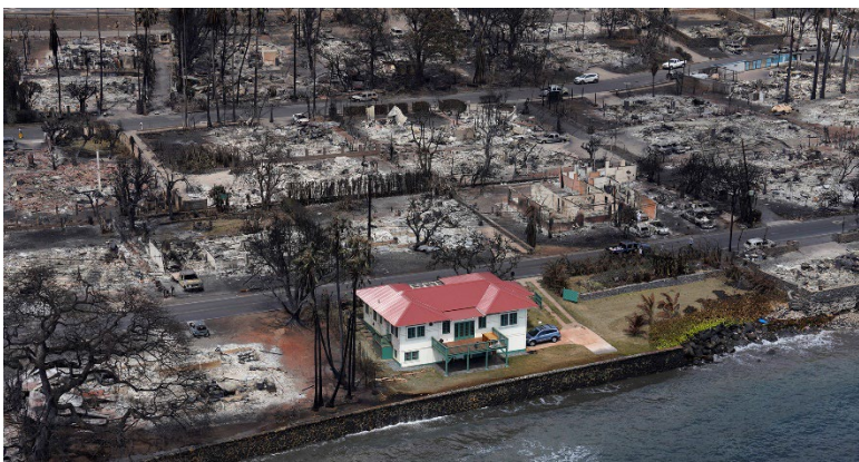
Figure 2-5: Aftermath of the Maui fires of August 2023, showing that some structures may survive in the midst of a fire blaze due to proactive measures taken by homeowners. Photo: Kevin Fujii/Civil Beat/2023, used under a commercial license, taken from https://www.civilbeat.org/2023/12/the-maui-fires-in-photos-august-2023/ .
