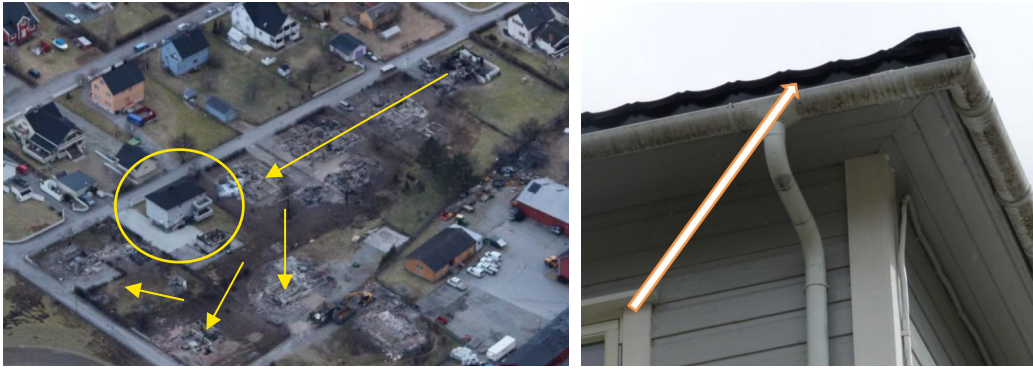
Figure 2-4: Left: Aftermath of the large fire in Lærdal of 2014, with yellow arrows showing the direction of fire spread, based on information of the fire spread in [21]. A yellow circle is added to mark the house that survived the fire. Right: This house had recently undergone renovations, in which cavities under the roof shingles were closed (arrow). Notice that the roof eaves are horizontal and closed, preventing embers from lodging. Left photo: Jan Christian Jerving, taken from NRK, https://www.nrk.no/vestland/to-ar-sidan-brannen-i-laerdal-1.12751469 , used with permission from photographer and NRK. Right photo: RISE Fire Research, taken from [21] with permission.
